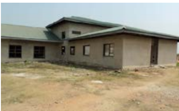
Plastering stage of the ECG office at Kentikrono, Kumasi
